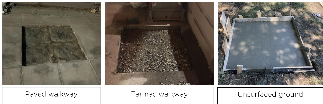
Figure 2.3 – Boundary conditions when laying the foundations.
