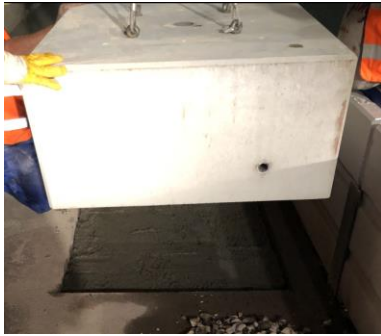
Figure 2.4 – Installation of the foundations.
