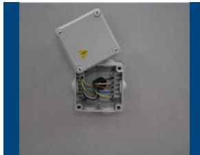
Waterproof terminal box IP-20. Caja de bornes estanca IP-20.
