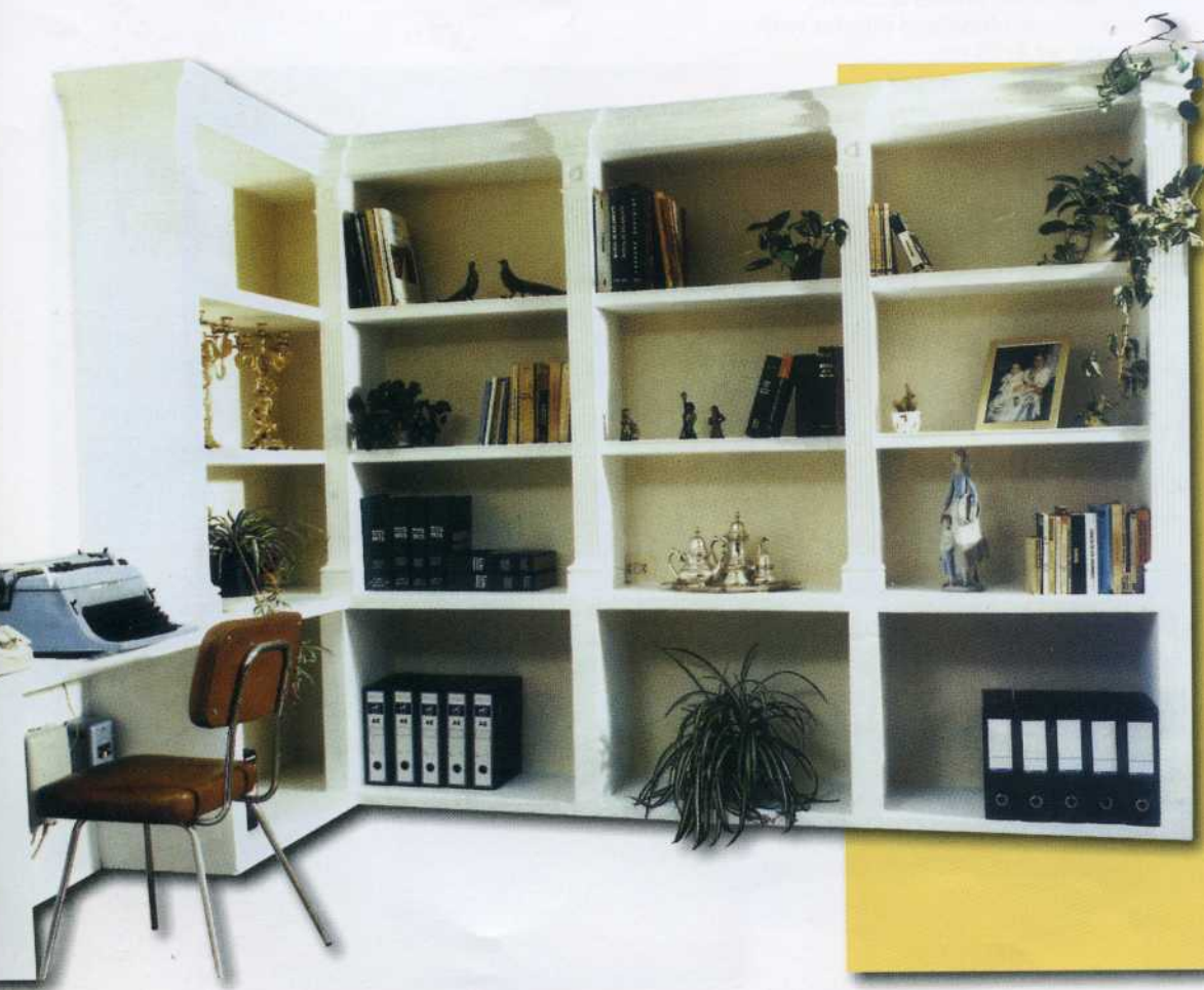
◀ Bookcase 3 Built with moulding shelves of 4x30x120, cornice capital of 11.5x21.3x8.7, pilasters with base and shelf friezes of 11.5x6.5x100
