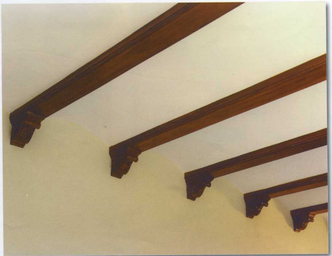
Mixed Ceiling ▶ Vaults Beams Corbels
